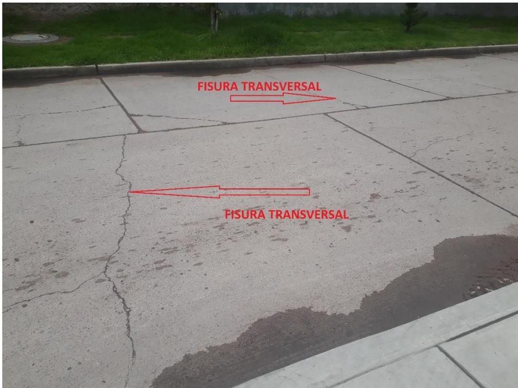
Figura 20: Fisura transversal o diagonal.
