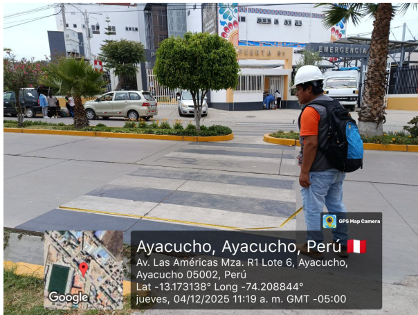
(a) Paso peatonal frente al Hospital Regional
