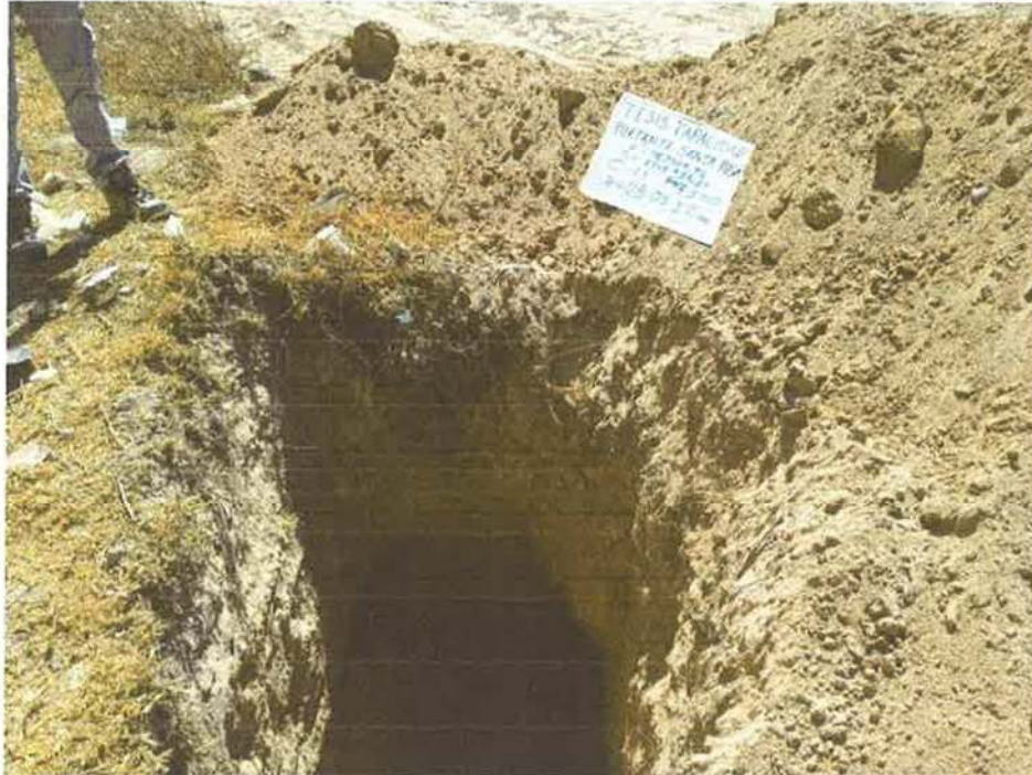
Figura 11. Calicata C – 11, Coordenadas 583505.96 E/ 8548936.81 N, Prof. 0.00 – 3.00 m
