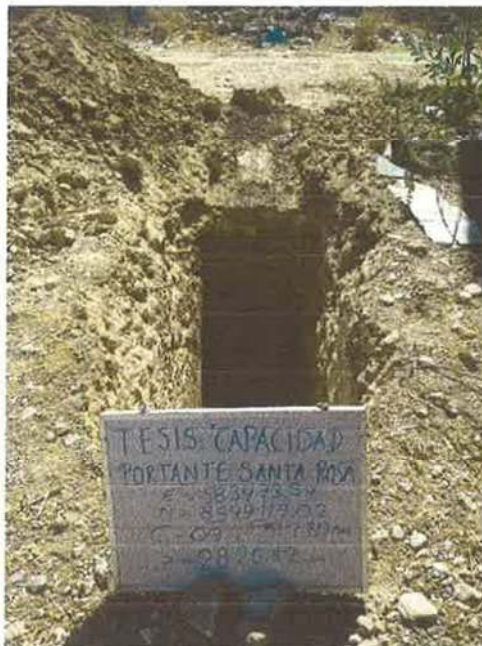
Figura 09. Calicata C – 09, Coordenadas 583473.54 E/ 8549119.02 N, Prof. 0.00 – 1.80 m
