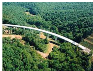
Figura 1.1. Puente Happy Hollow, Tennessee, USA
